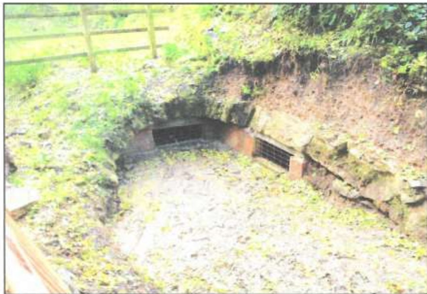
Completed wheelpit site
