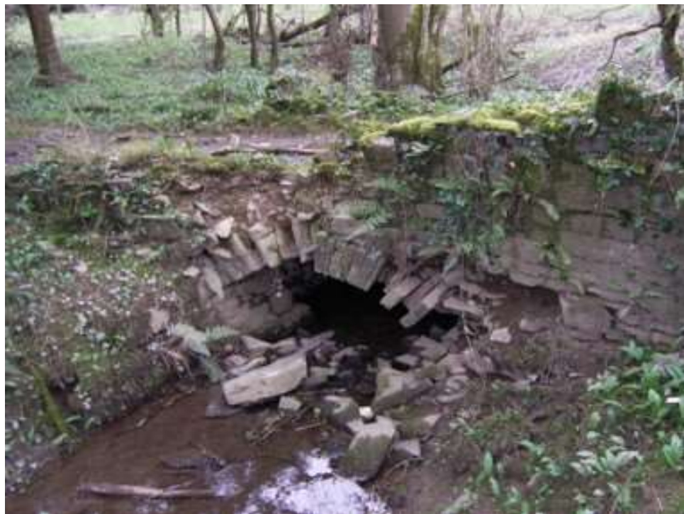
Tucking mill exit channel
