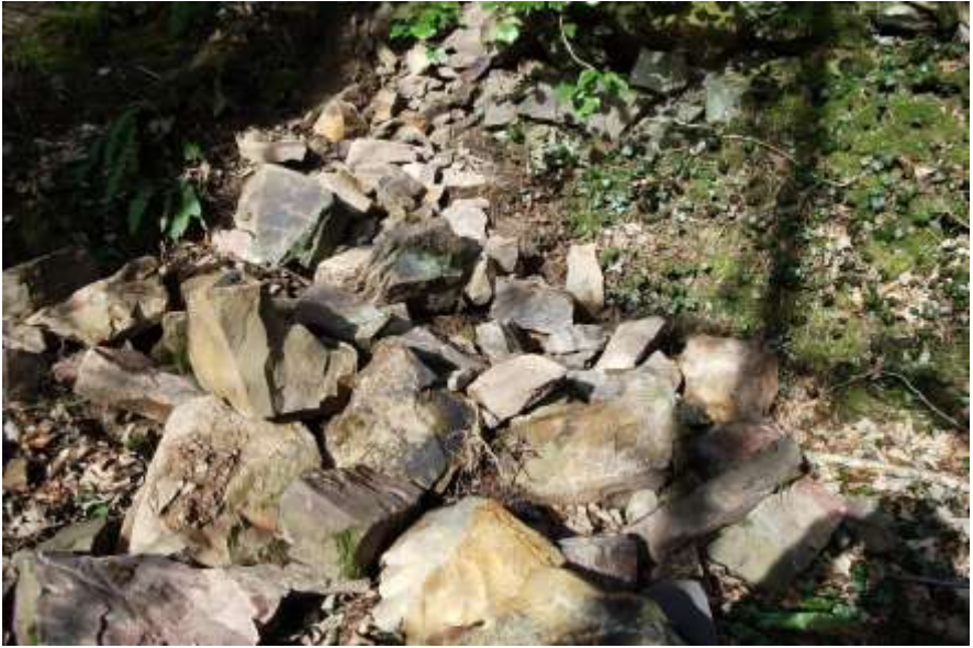
Picture above shows stonework fallen from one of the major revetments, following the effects of two hard winters Tony Barnes 2012
